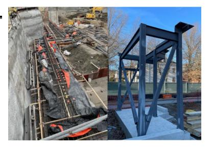
New Drain Line installed and has been connected to the Tannery Brook line, the drain line that used to run through the middle of the site has been removed.
